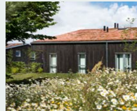
R03 TØMMERGÅRDEN BUILT 2016 531 m 2 1 - 2 STOREYS 19 OCCUPANTS
