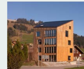
E07 SOLARHOUSE BUILT 2014 536 m 2 5 STOREYS 5,5 - 12 OCCUPANTS (INTERNATIONAL CASE)
