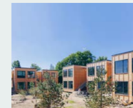
E08 CPH VILLAGE VESTERBRO BUILT 2020 154 m 2 2 STOREYS 8 OCCUPANTS
