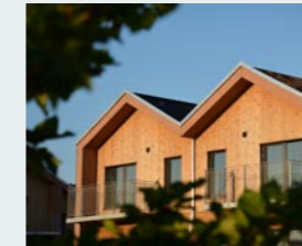
E02 TANKEFULD II BUILT 2020 2853 m 2 2 STOREYS 128 OCCUPANTS
