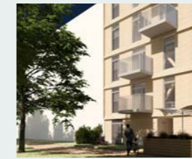
E01 MINICO2 MULTI-STOREY TIMBER IN PROGRESS (2023) 579 m 2 5 STOREYS 18 OCCUPANTS
